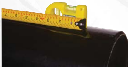
Level pipe for fit up
